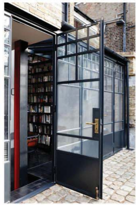
This side and rear extension features Crittall steel-glazed windows and doors. The British firm is the original maker of this type of window, which has an industrial yet Art Deco look
