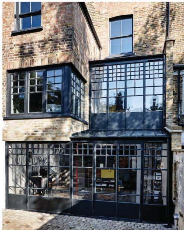
This side and rear extension features Crittall steel-glazed windows and doors. The British firm is the original maker of this type of window, which has an industrial yet Art Deco look
